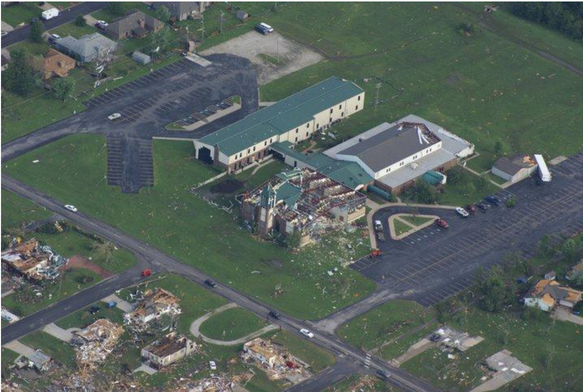
Photo 7: Saint Paul's United Method Church Complex constructed of multi-pre-engineered metal buildings.
