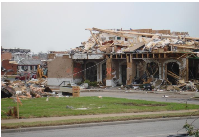
Photo 5: Non-residential building remains standing despite major damage.
