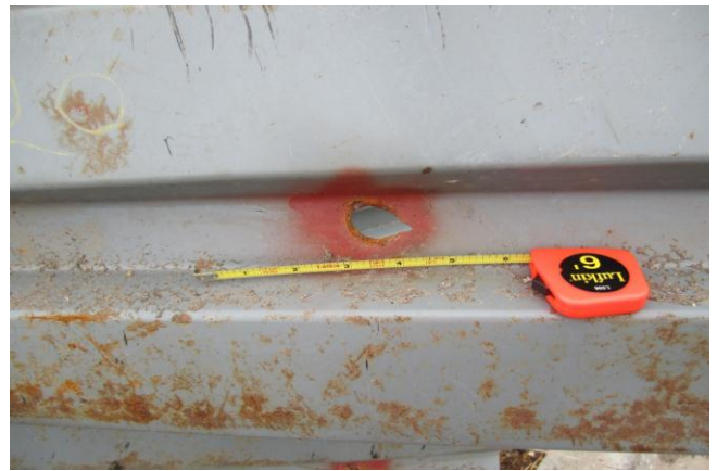
Photo 27: Embed plate with short studs pulled free from top of CMU wall.
