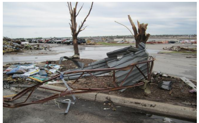
Photo 31: Both metal deck and steel joist blown clear from building footprint.
