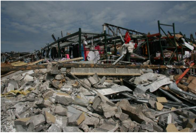
Photo 26: Roof level bond beam detached from top of CMU wall.
