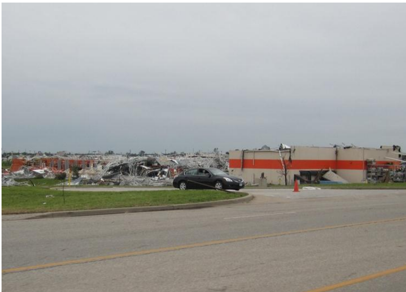
Photo 25: This is one example of a hard wall building system struck by the Joplin Tornado. It is noted that some walls remained standing due to a true cantilever condition of the tilt-up wall panels being support at their base and attached approximately four feet above, at a loading dock slab.
