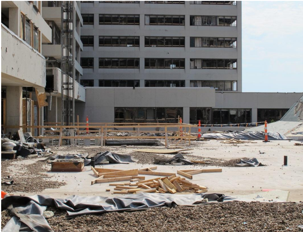
Photo 13: Concrete-frame building at left, steel frame building beyond.
