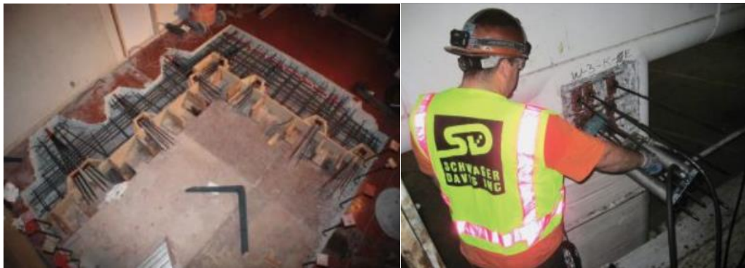
Figure 3: Post-tensioned slab opening for repair. Figure 4: Tendon being re-stressed after repair.
