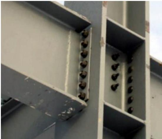
**Figure 1:** Steel Moment Connection
