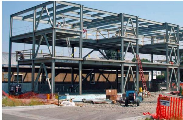
**Figure 5:** Braced Frame
