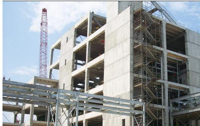
**Figure 3: Concrete Shear Walls**
